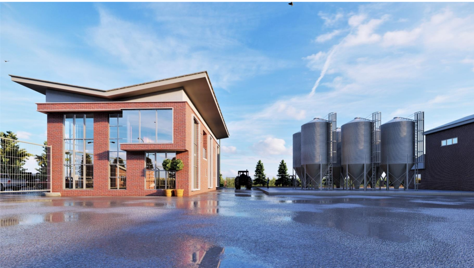
ADMINISTATIVE BUILDING & SILOS
