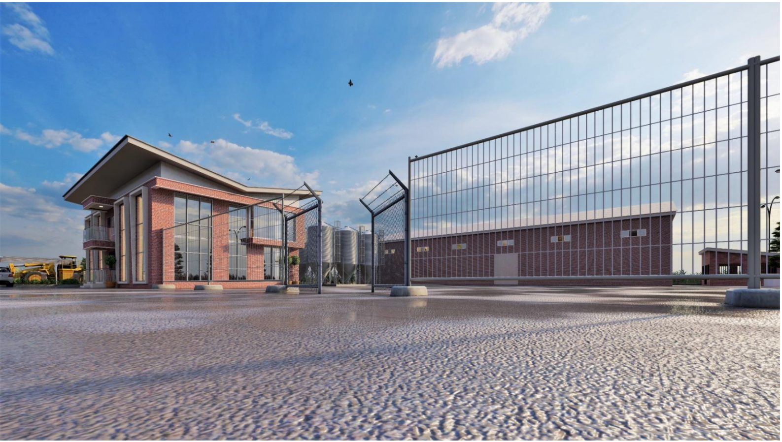
FACTORY & ADMINISTATIVE BUILDING
